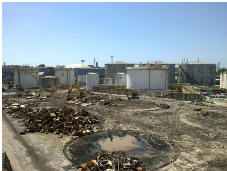
Area ripulita dai racks e piping.
